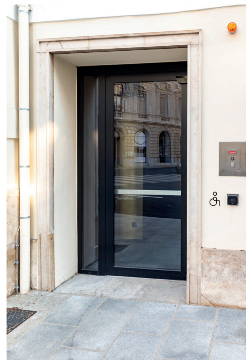
Accessible side entrance
