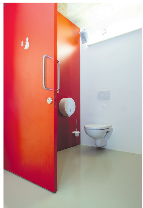
Low-barrier WC in the basement
