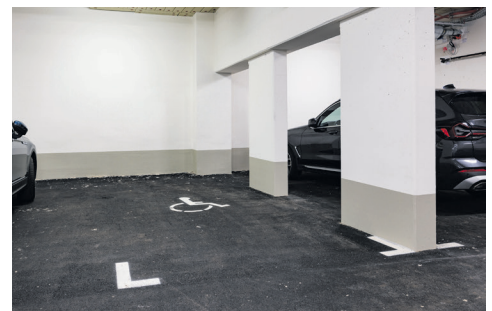
Barrier-free car park
