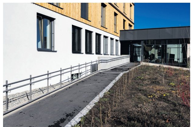
Ramp to barrier-free entrance
